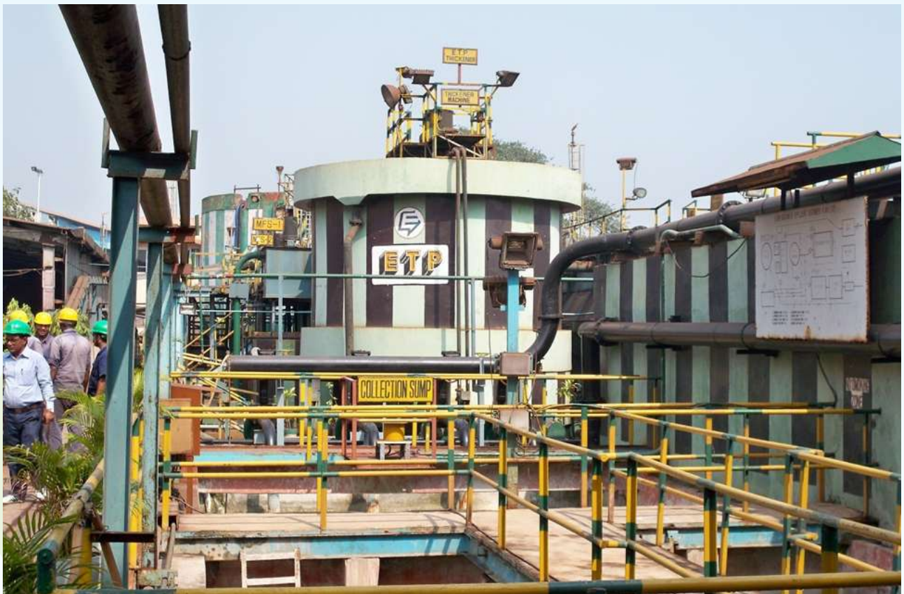
Figure 3 - Common Effluent treatment plant at Khardah
