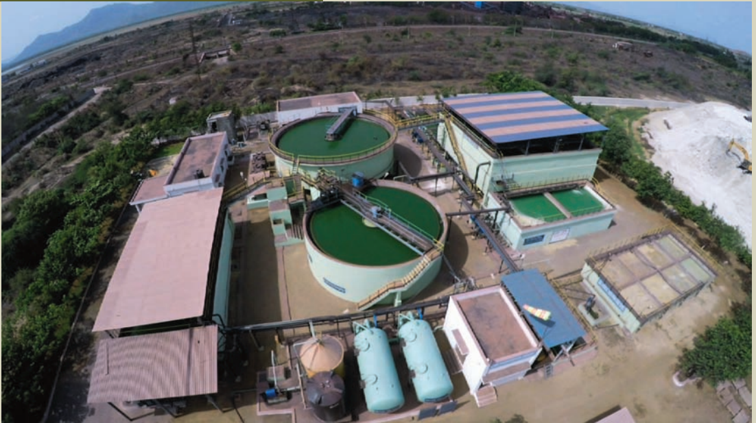
Aerial view of the Water Treatment Plant where Tirupati Municipal Sewage Water conveyed through pipelines is treated for Industrial use, an initiative first of its kind in the State to conserve ground water
