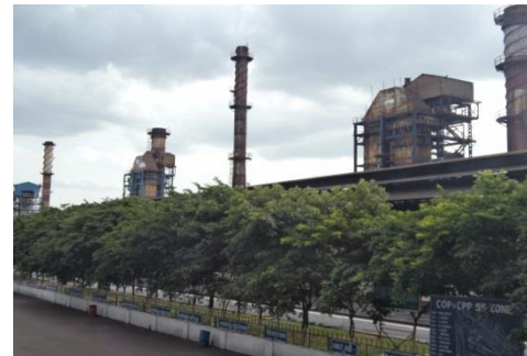
Power Plant: 12 MW & 2.5 MW
